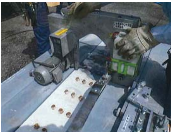
(b) Cutting of studs on main girder
