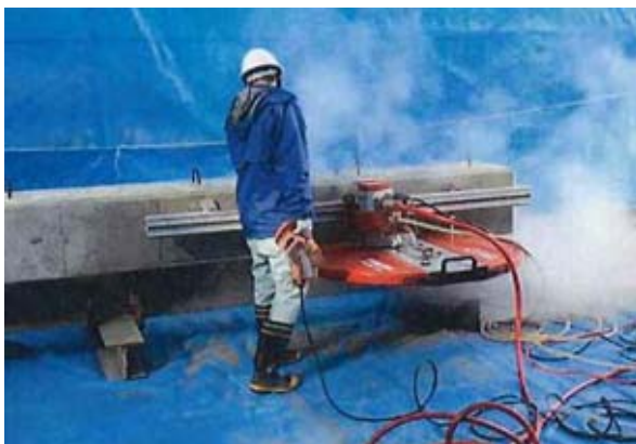
(a) Horizontal cutting of concrete blocks on main girder
