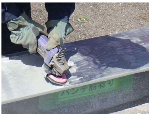
(c) Surfacing with spark disk
