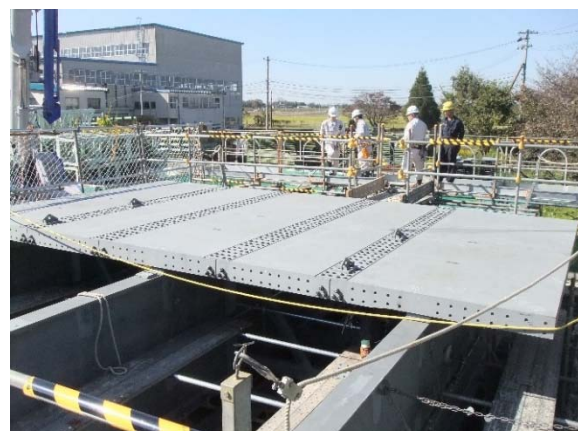
(b) Erection of slab members
