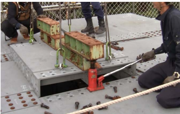
Figure 10. Removing a slab using a jack
