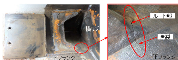
(c) CP切欠き部のき裂
